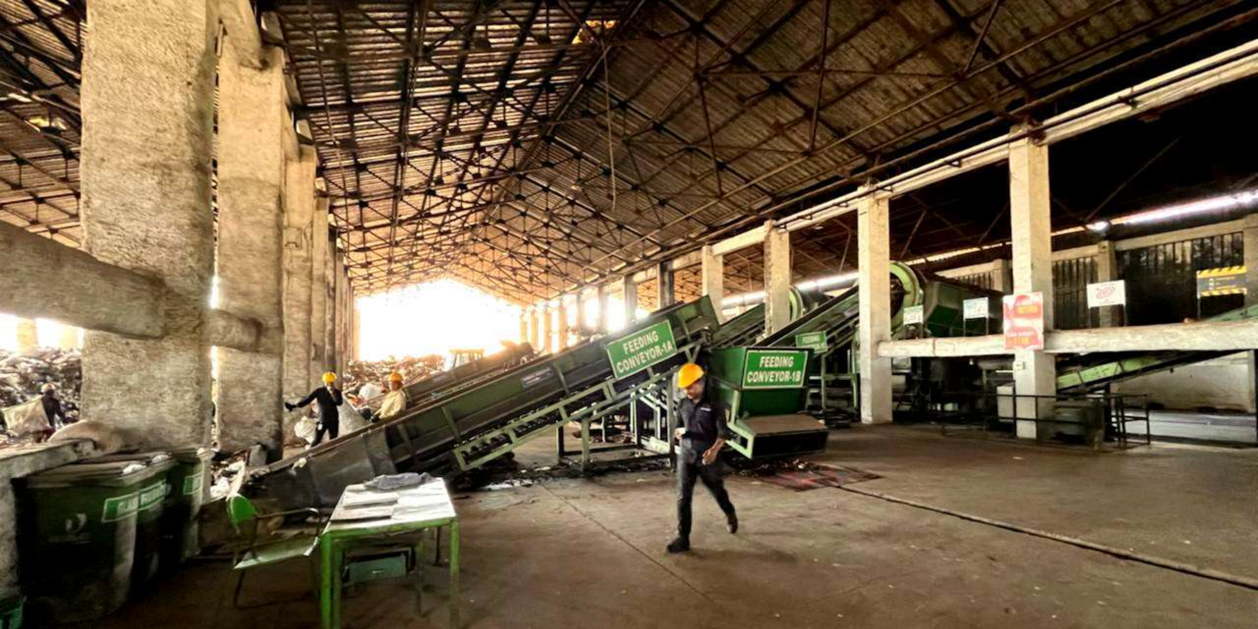
MRF facility at Moshi Garbage Depo
