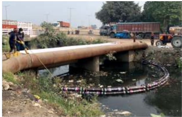
Boom Barrier in Action
