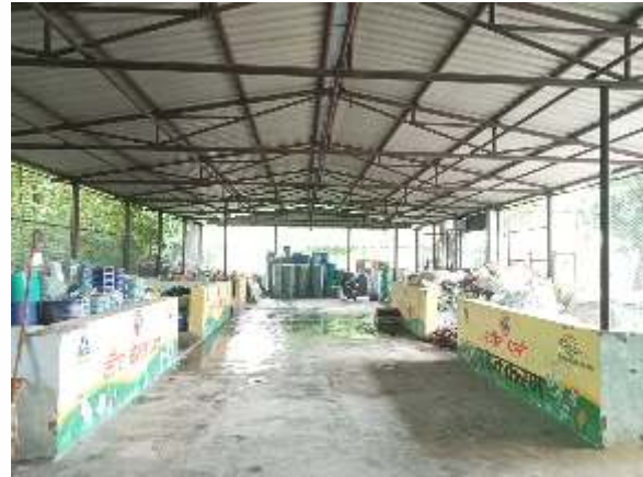
Material Recovery Facility Centre
