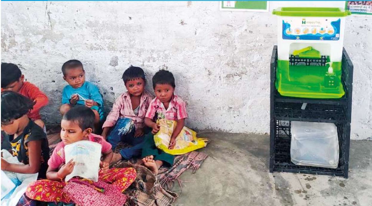
Figure 40: HappyTaps prototype installed in the Anganwadi centre, Rajpur block, Hathras
