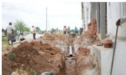
Fig: Simplified Sewer System
