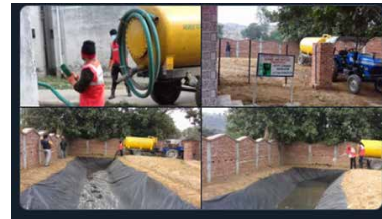
Figure 6: Faecal Sludge Treatment Plant in Chunar under construction
