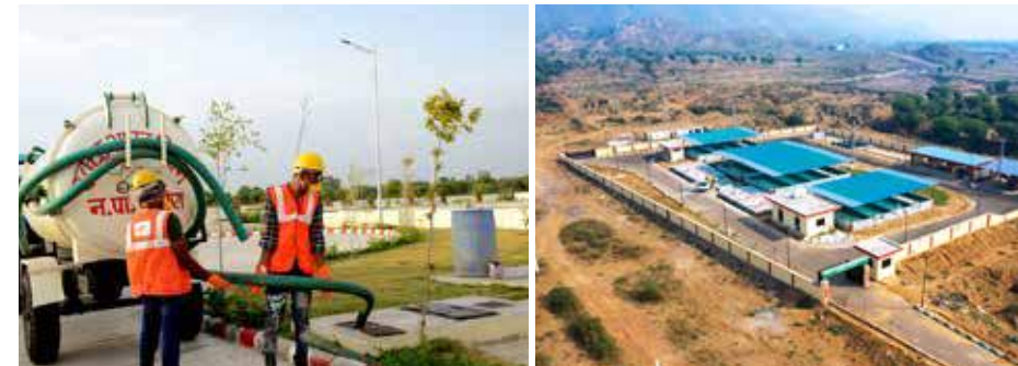
Figure 5 & 6: Constructed and Operational FSTPs in Rajasthan
