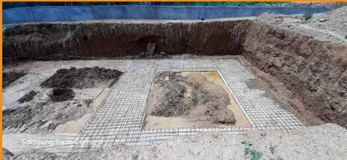
Figure 5: Faecal Sludge Treatment Plant in Chunar under construction
