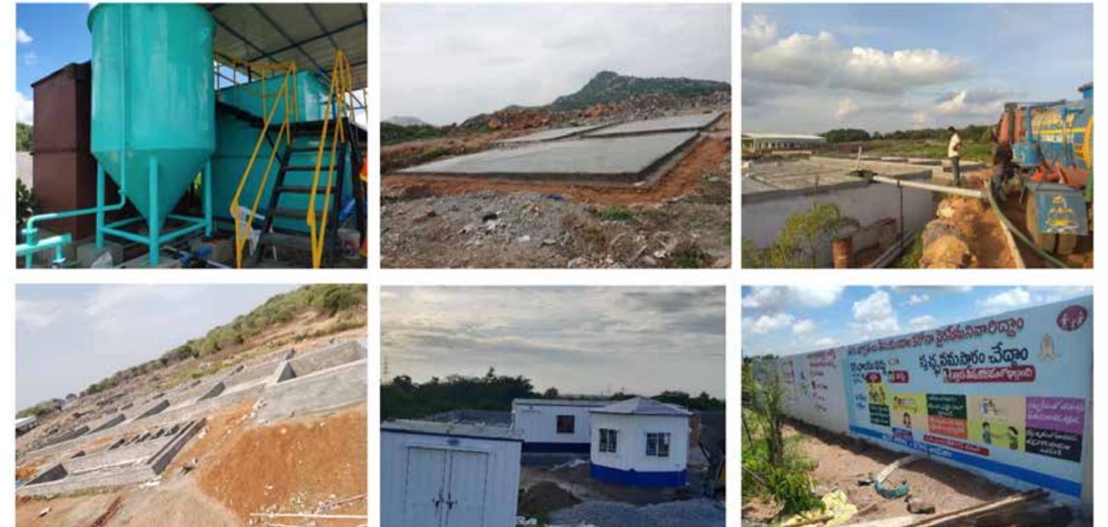
Figure 5: FSTPs in different states of construction in ULBs in Telangana
