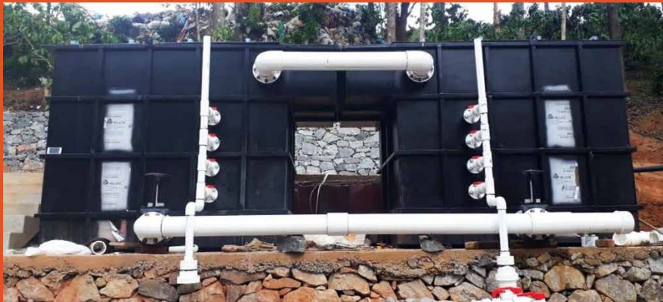
Solid-Liquid Separation Tank
