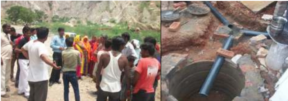
Figure 6: ; Training of masons in twin pit toilet technique
