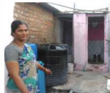
Figure 4: Archana has constructed a toilet and bathroom with plastering and tiling. Access cover for opening the septic tank is also properly placed. Cost of construction of the toilet was approx. Rs 50,000. She has borrowed Rs 11,000 from ICICI bank
